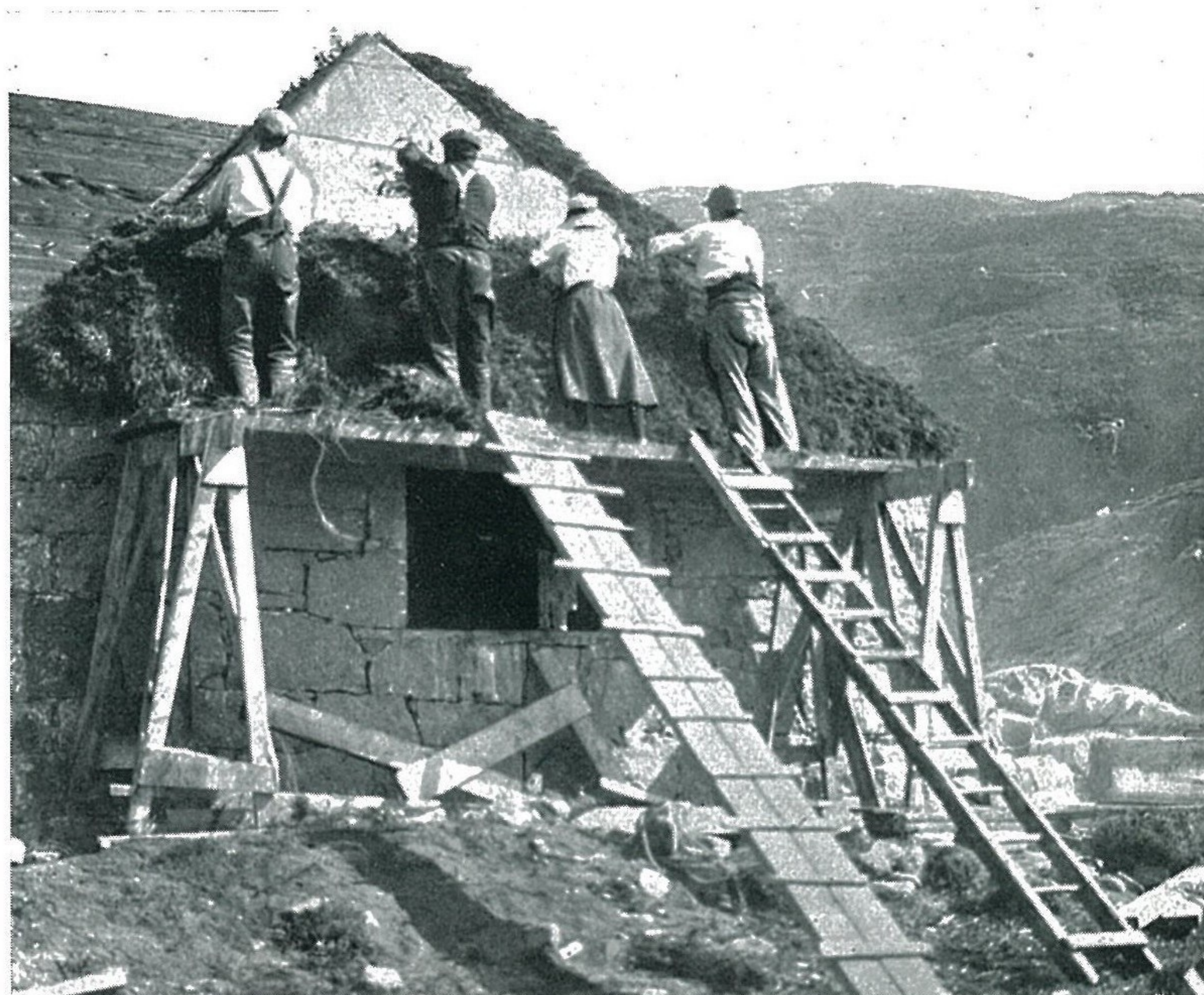
THATCHING IN PROGRESS, THE WRITER (THIRD FROM LEFT) ASSISTING.
