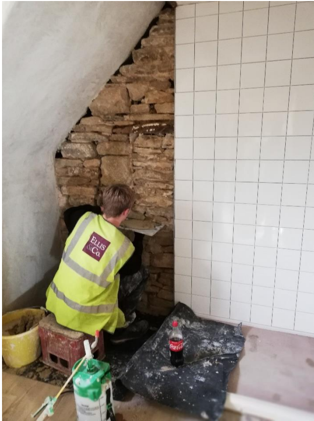
Careful repointing in lime mortar.
